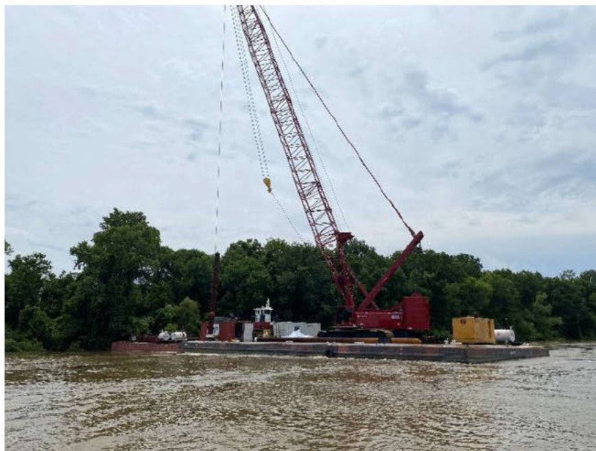
Figure 2. Crane barge and Flexifloat along the east bank. (June 16, 2023/Sector Mobile IO)
